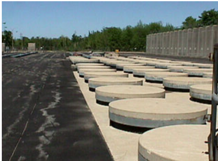
Figure 5: In-ground containers used to store ILW at the WWMF
